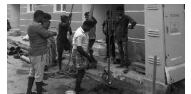
Men installing pumps to lift ground water | JOSEPH SEBASTIAN
