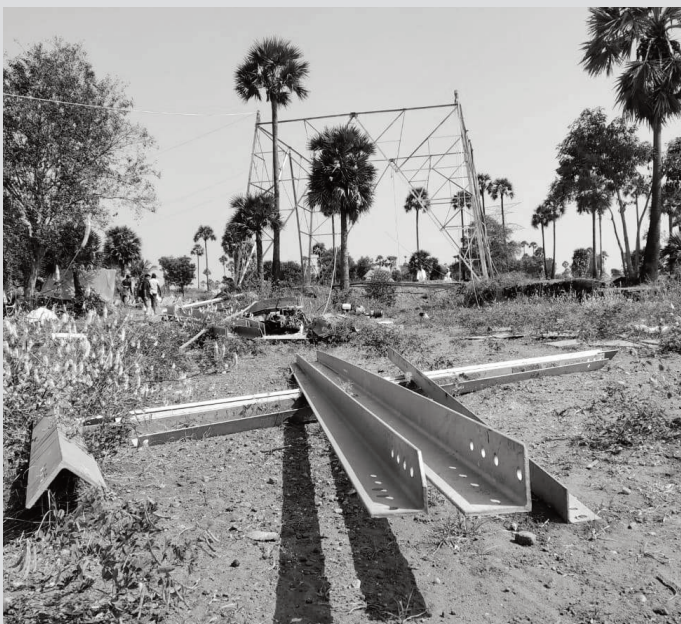
Steel plates for separating tiers of a tower | ANUSHKA DEEPAK
