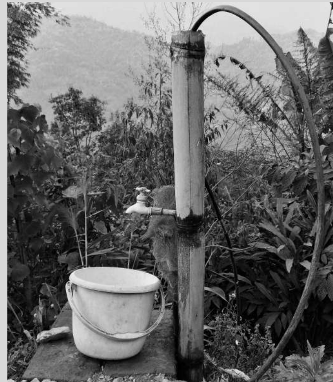
Pipes are often inserted into hollow bamboo logs with an attached tap to fill buckets or pitchers | MUSKAAN SHARMA
