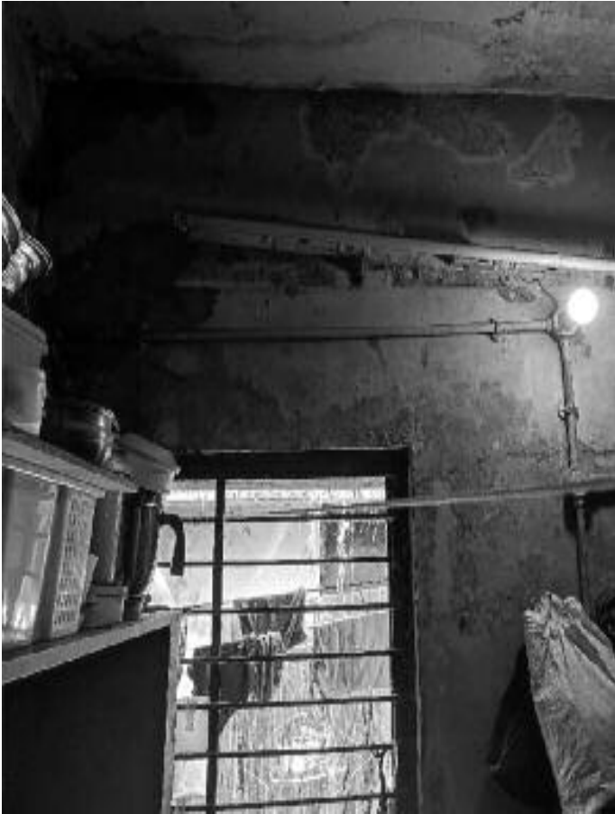
Plaster peeling off in a house | PHOTO: SHAURYA SINGH THAPA
